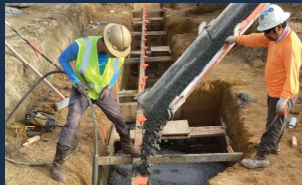
Concrete footings are poured
