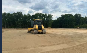
Site is graded & compacted
