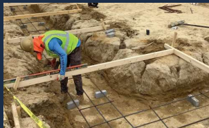
Footing holes are prepared
