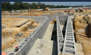
Foundation walls are started
